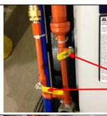
Make sure the air control valves on the INJECT-AIR are in fully closed position.
